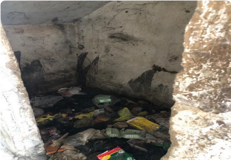
Plate 1: Blocked Drainage by Solid Waste in Zoo Road Estate, Kano, Nigeria Source: Researcher's field work 2025
