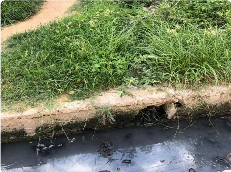
Plate 2: Stagnant drain water due to Drainage blockage, Zoo Road Estate, Kano Source: Researcher's field work 2025
